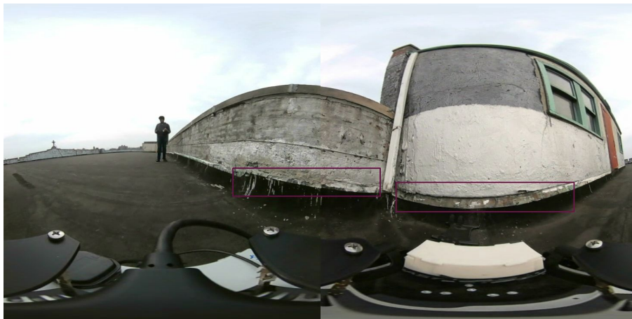
Figure 4.1: Base Flashing-Coated Metal
