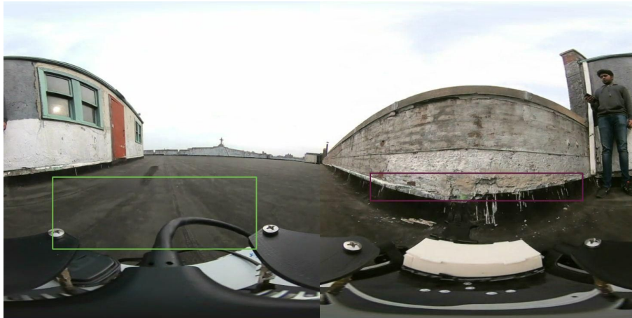
Figure 4.3: Base Flashing-Membrane Material
